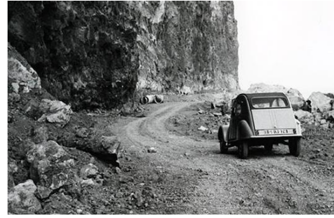
Construction de la route littorale - 1963
